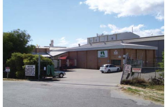
Entrance to the Kwinana manufacturing plant
