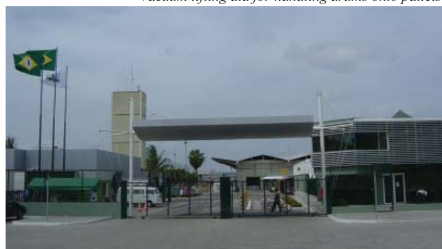
The main entrance to the site has been improved to give better control and security for people and transports
