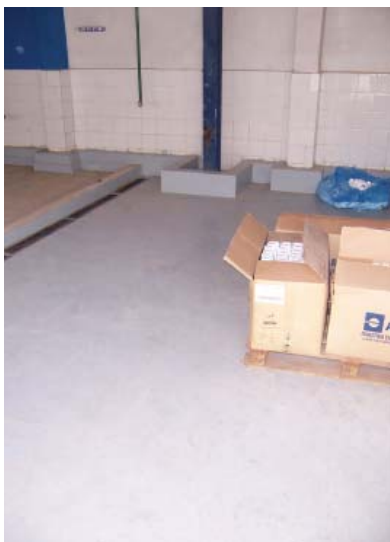
A3 floor replacement
