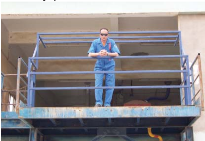
Safety cage for loading materials
