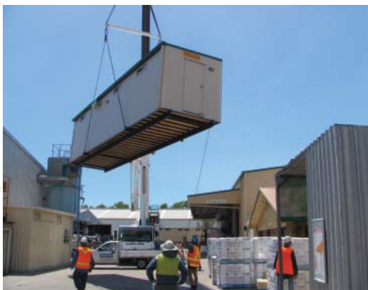
Lifting the new amenities block into position
