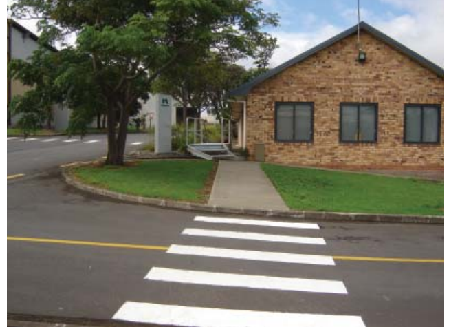
Pedestrian walkways have been designated to separate them from vehicular traffic
